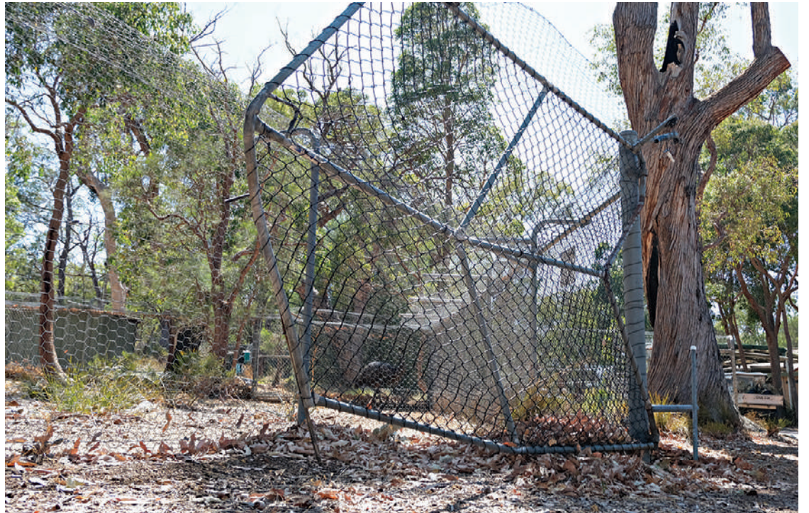
One of the destroyed gates is right next to the emu enclosure. Picture: Andrew Williams
