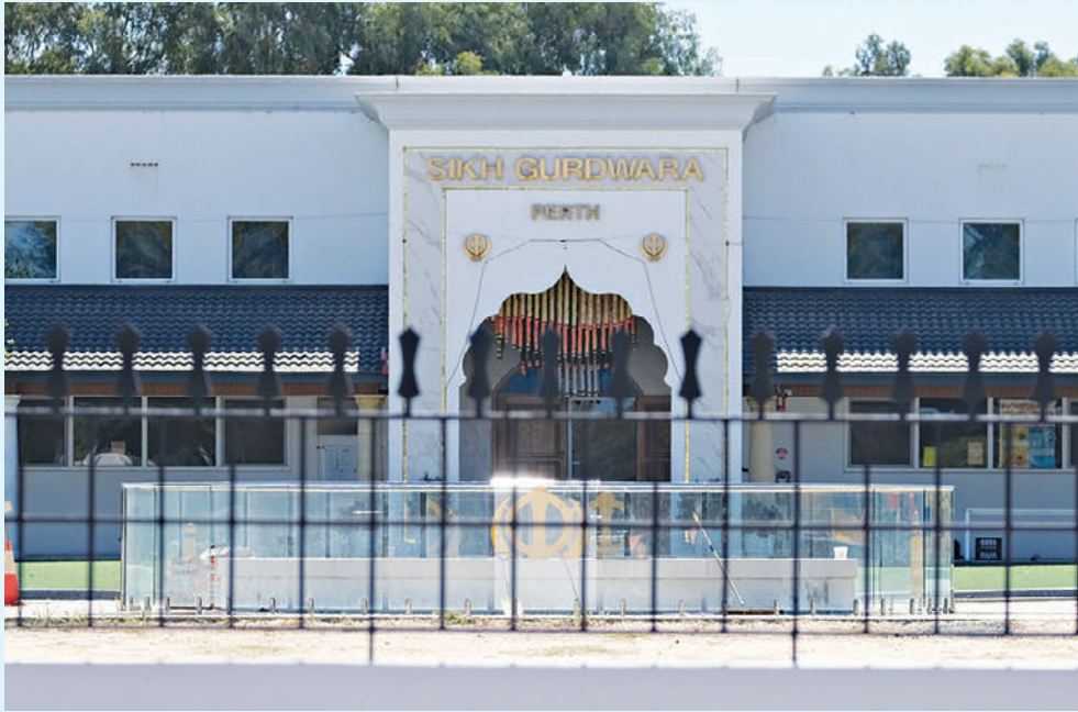
The Sikh Gurdwara in Bennett Springs has been awarded $250,000 to undertake sewer and water projects. Picture: Andrew Williams
