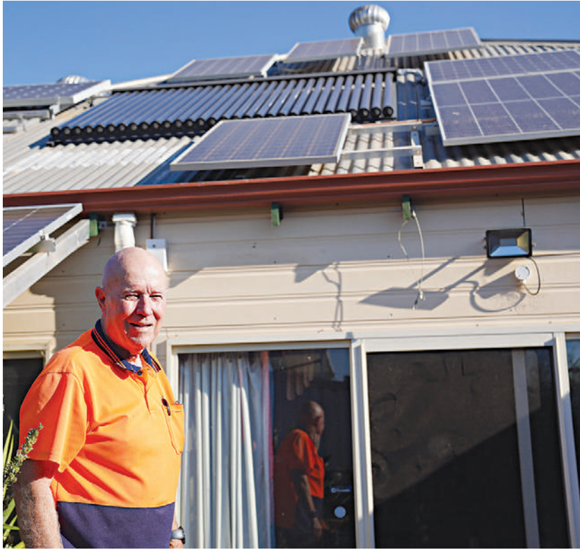
Martin Chape and his solar panel array. Pictures: Guanhao Cheng
