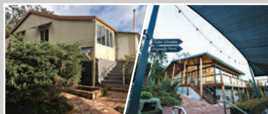
Core Cider House Before and After
