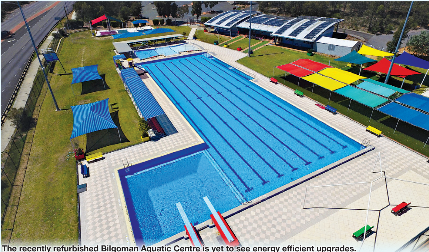
The recently refurbished Bilgoman Aquatic Centre is yet to see energy efficient upgrades.
