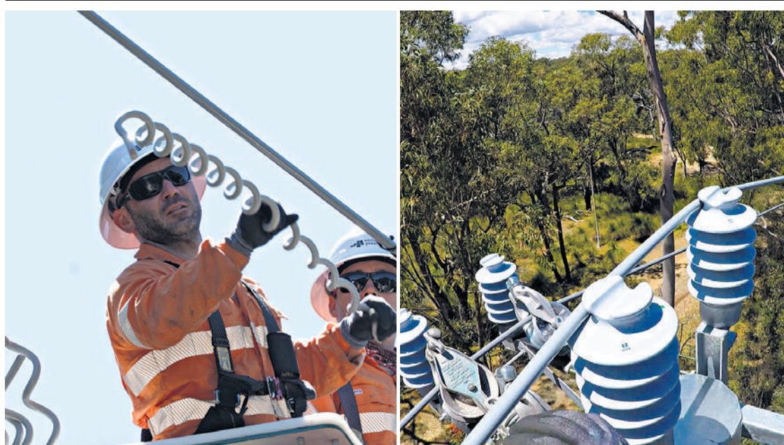
Western Power crew install covered conductors. Covered conductors to be installed in Parkerville. Pictures: Western Power.
