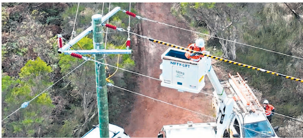
Western Power has been installing bird diverters to protect fauna.
