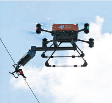
Drone Installation of a bird diverter. Picture: Western Power.
