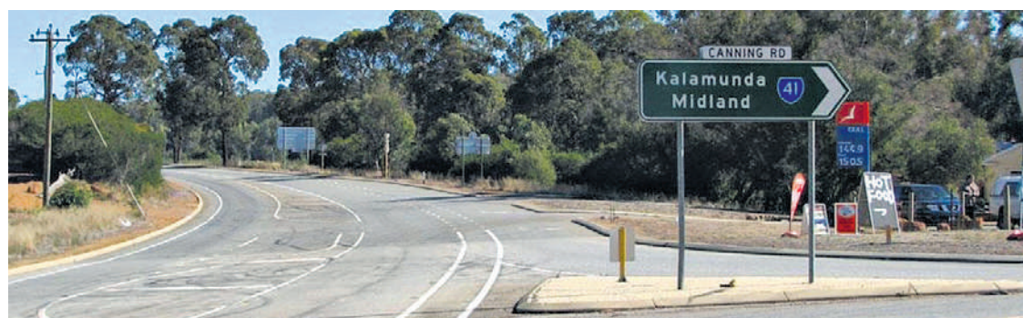
Canning Road is among the routes proposed for upgrades as part of a $5 million funding submission by the City of Kalamunda. Picture: Supplied
