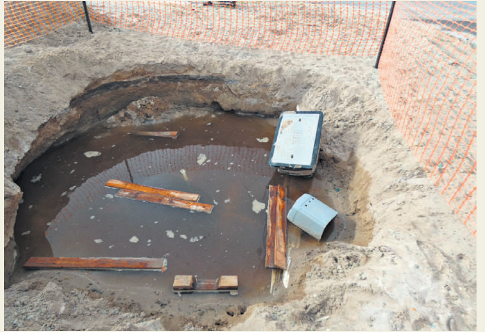
Development in Dayton where high groundwater submerges an NBN box.
