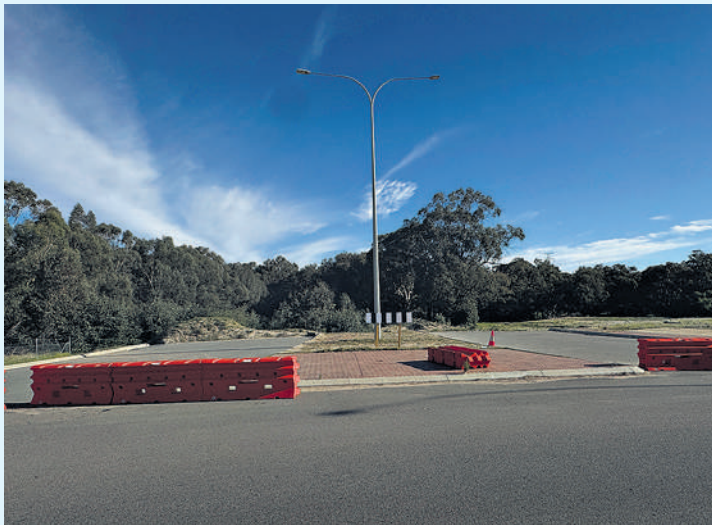
Barriers remain in place at the proposed Lloyd Street bridge extension site. Picture: Daniel Holmes
