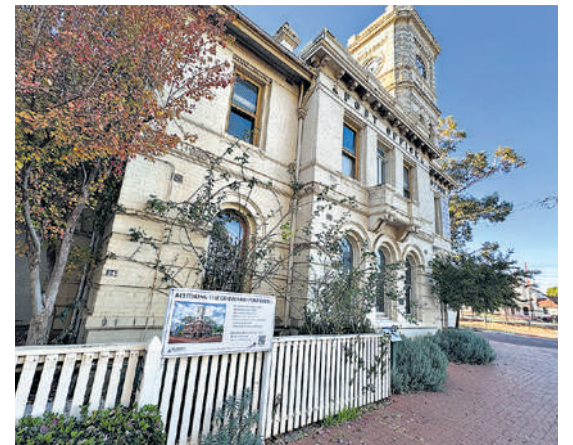
A takeaway coffee window and patisserie is planned for the north side of the building. Picture: Brayden Mould
