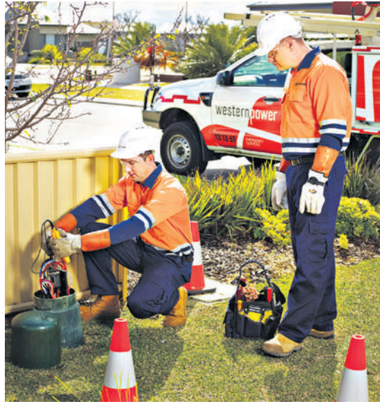
Town of Bassendean is progressing an agreement with Western Power to move power underground in Bassendean North. Picture: Western Power
