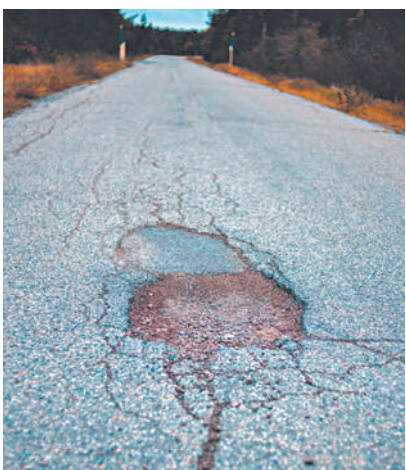
A jet paver will begin working on fixing potholes in Toodyay from July 20.
