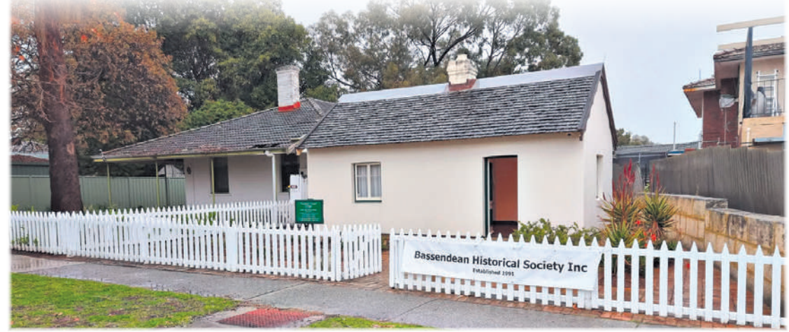
The cottage is recognised by heritage registers and regarded as the oldest surviving building in Bassendean. Picture: Bassendean Historical Society
