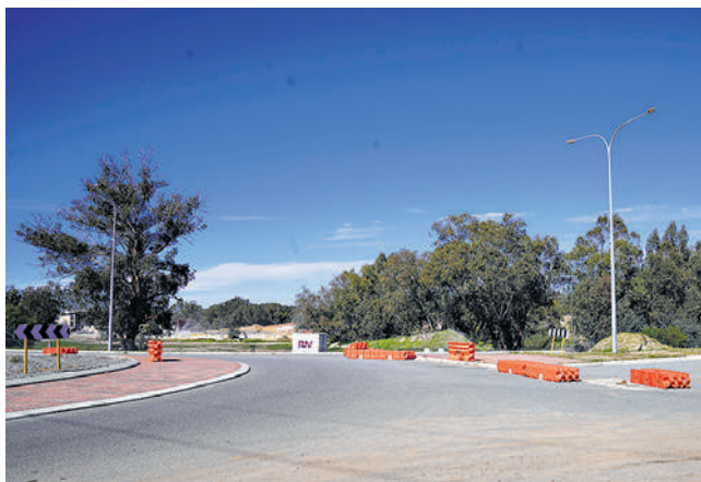
A part of Lloyd Street to be connected by the bridge.
