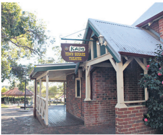
The KADS theatre in Kalamunda had been subject to vandalism prior to the program's start. Picture: Camila Egusquiza Santa Cruz
