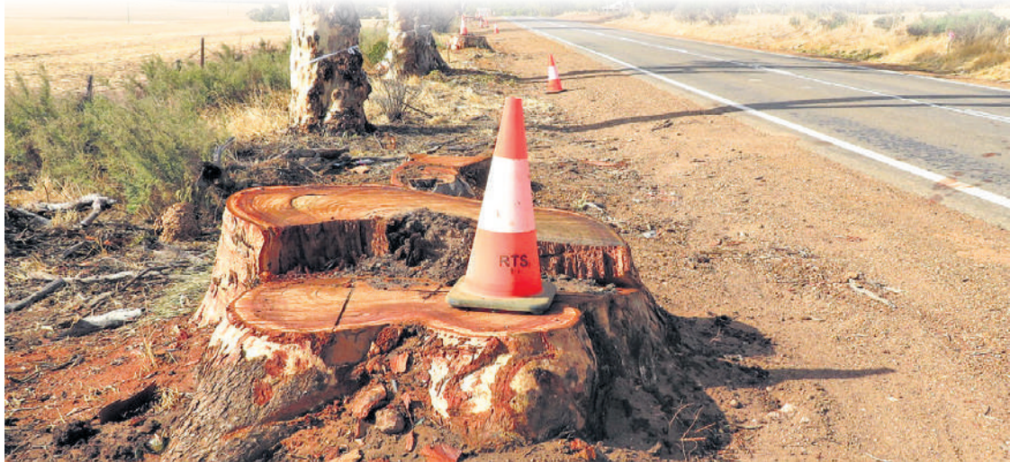
Mature tree stump left from clearing done for the Northam-Pithara Road widening project. Picture: Brett Loney
