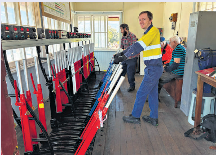
The signal cabin will be one of only two operational signal cabins in WA.
